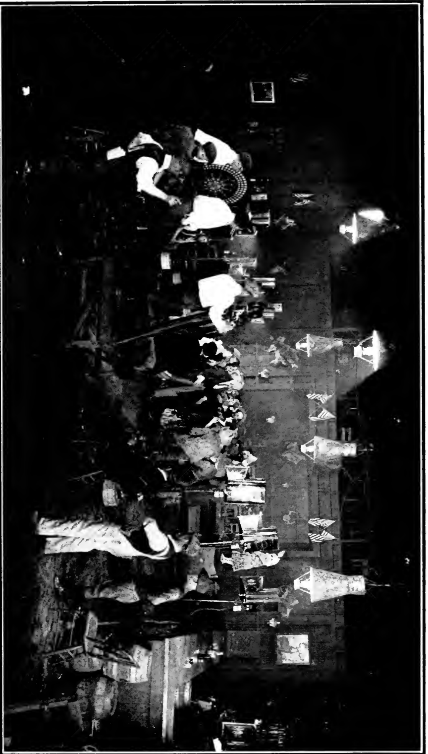
(Courtesy Robertson-Cole Productions) STUDIO USING ALL "HARDY" OR ARC LIGHTS. OVERHEAD LIGHTING FROM DOMES. IN THIS SET THE DOMES SERVE A DOUBLE PURPOSE BEING CANOUPED WITH OIL LAMPS FROM WHICH THE LIGHT APPEARS TO COME.
